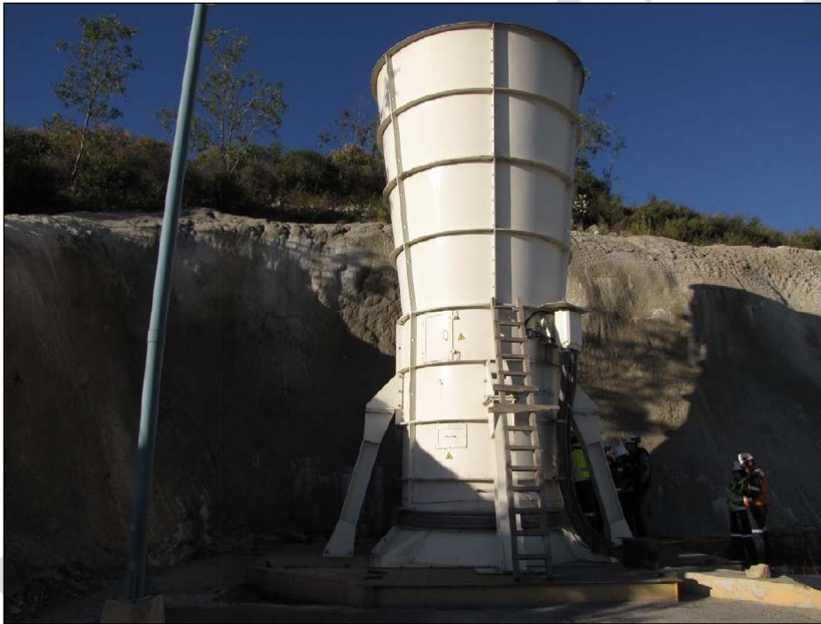
Figure 62: Rosarios Main Exhaust Fan (FSM 2017)
