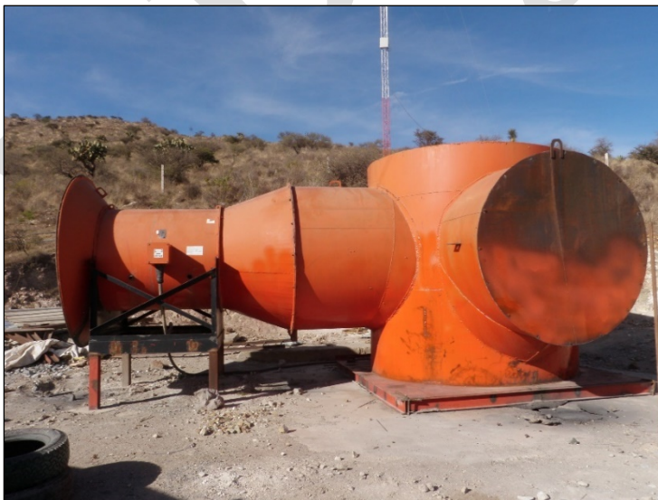
Figure 64: Quebradillas Exhaust Fan (SRK 2017)
