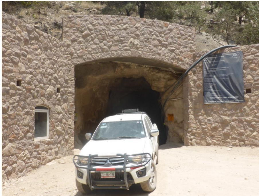
Figure 16-33: Perseverancia Mine: Main Portal
