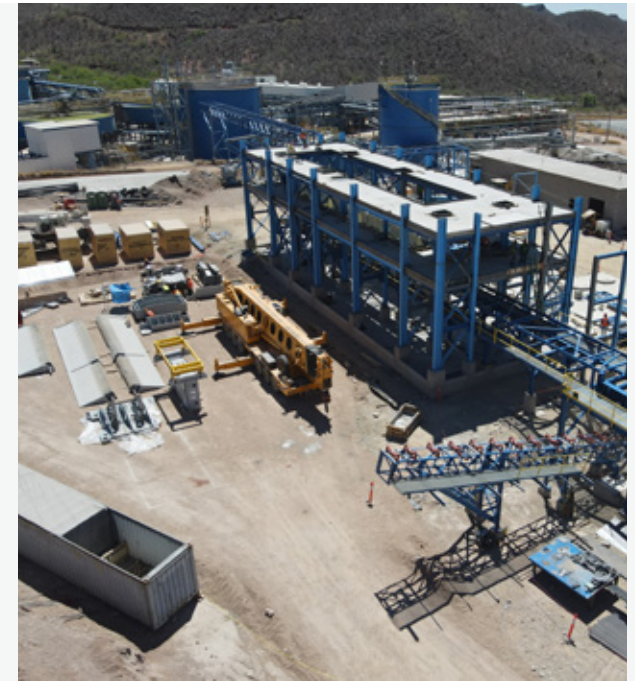
TAILINGS FILTER PRESS CONSTRUCTION IN SANTA ELENA
