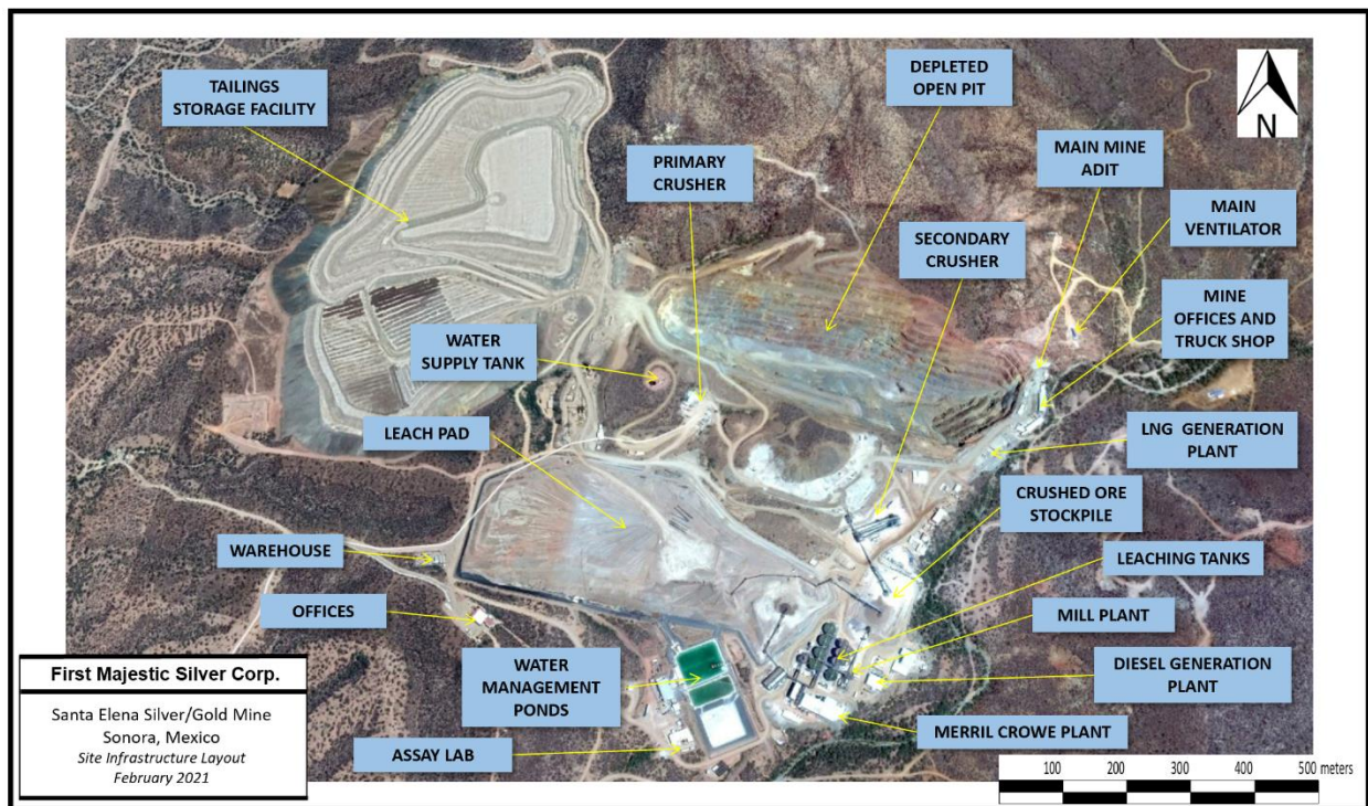
Figure 18-1: Santa Elena Mine Infrastructure
