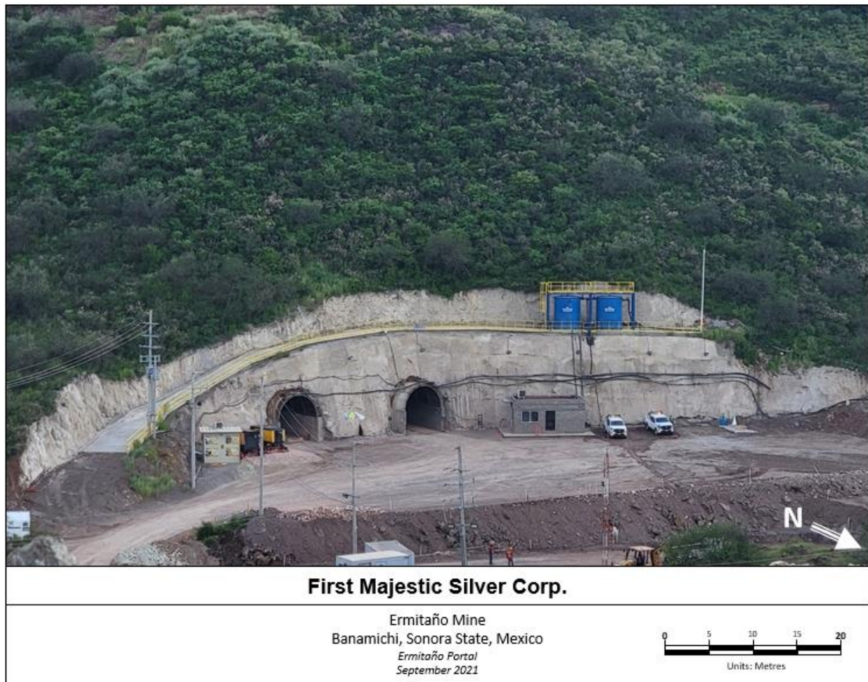
Figure 16-32: Ermitaño Mine Portal
