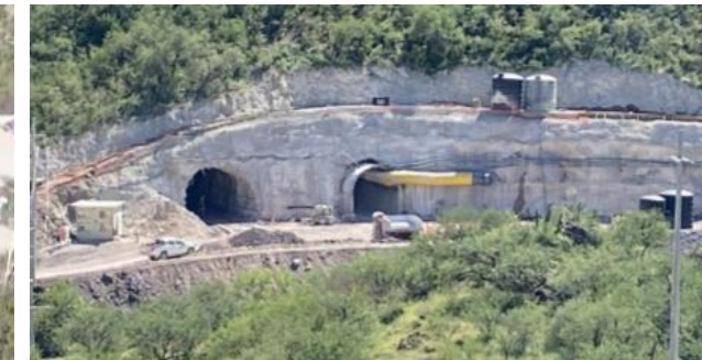
Ermitaño East & West Portal
