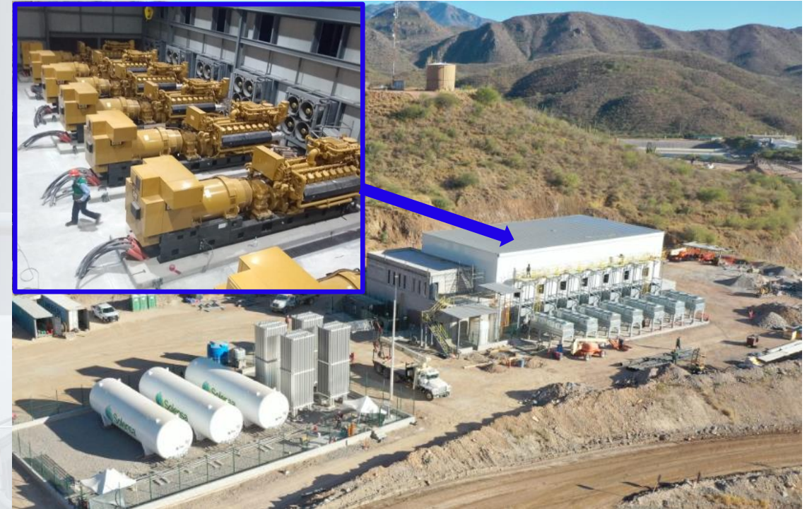
Santa Elena's new 12.4MW LNG Power Plant
