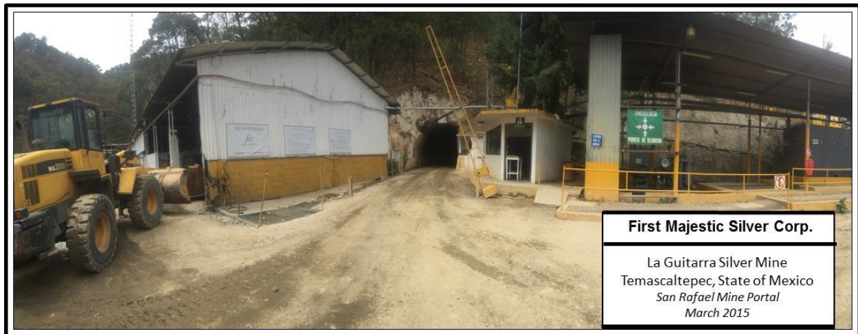
Figure 18-2: Image of the San Rafael mine portal
