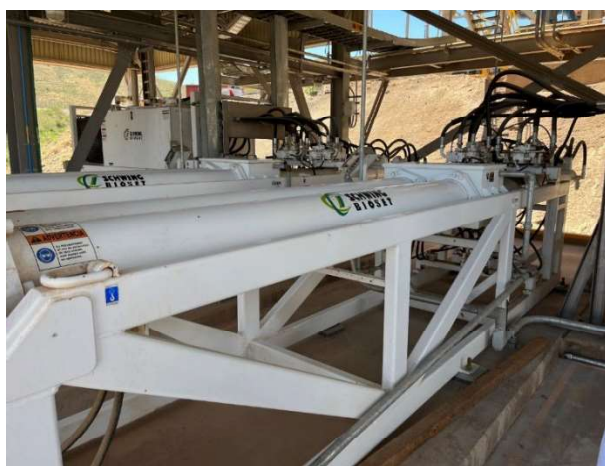
Figure 18.10: Tailings Dewatering Disc Filter (left) and Positive Displacement Pumps for Paste Fill (right)
