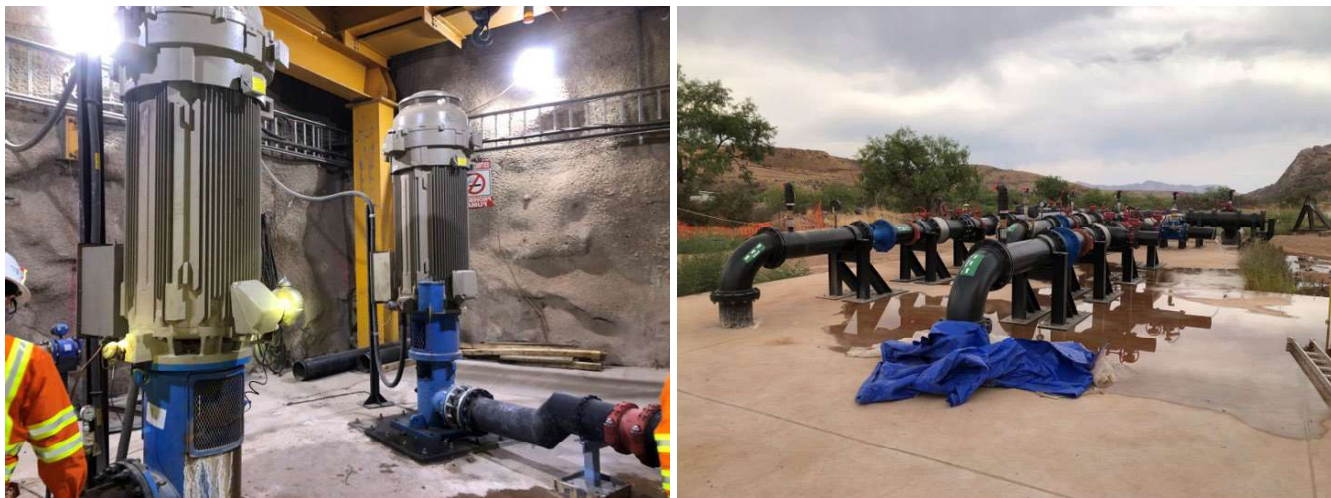
Figure 18.8: Underground Wellhead Pumps and Surface Discharge Header
