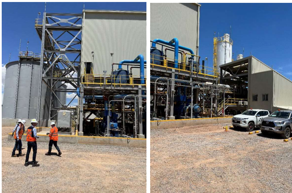
Figure 18.9: Filter Feed Tanks (left), Vacuum Pump, and Binder Silo (right) at the Paste Fill Plant
