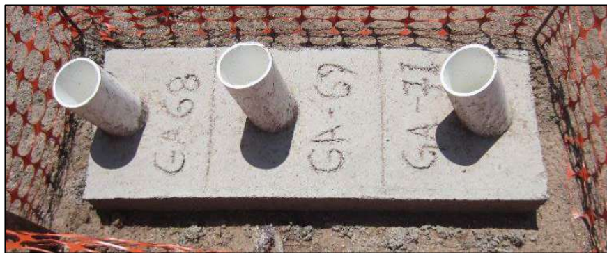
Figure 10.5: Example of a Completed Drill Hole Site
