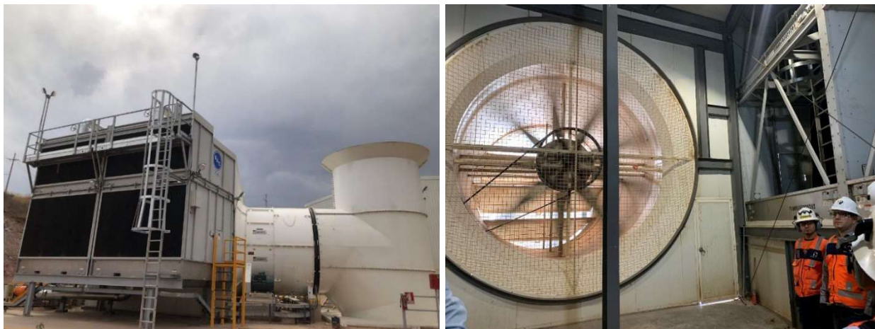
Figure 18.7: (A) Air Intake through Bulk Air Cooler and Delivery to Underground by Injection Fan (B) Injection Air Fan at Refrigeration Plant 1
