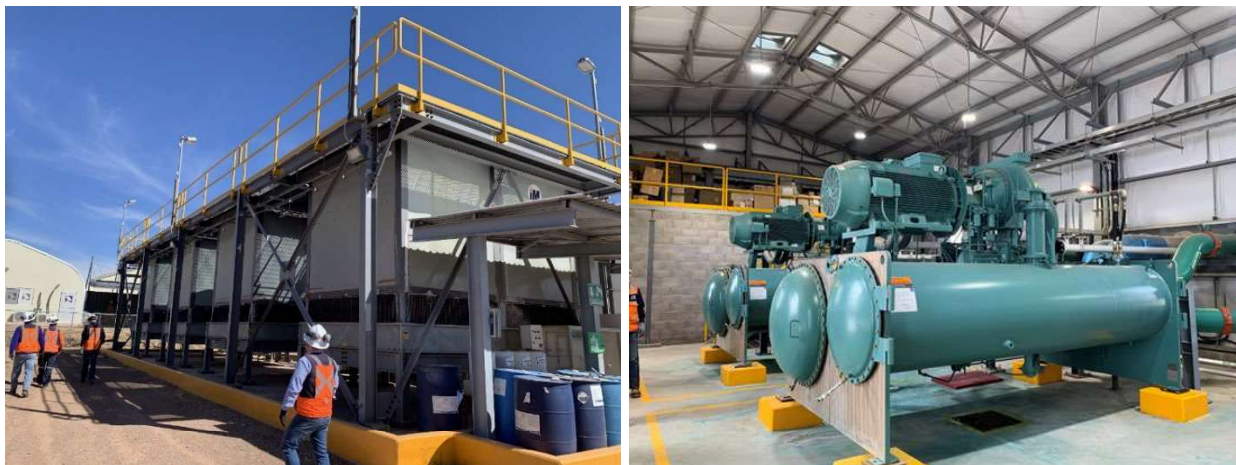
Figure 18.6: (A) Evaporative Cooling Towers as the First Stage of Cooling (B) Mechanical Refrigeration Units at Refrigeration Plant 1 as Second Stage of Cooling
